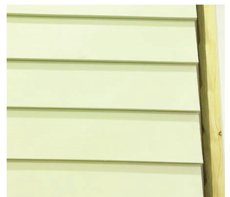
Nail fixing onto timber studs
