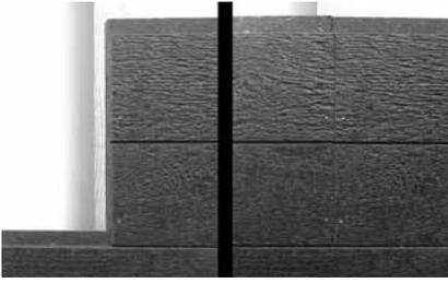
Selflok Weatherboards may also be mitred at 45° and joined on stud.
