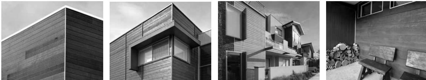
**Note:** Natural Products are composed of unsealed natural hardwood timber which may occasionally exhibit tannin bleeding. Consideration must be taken if installing unsealed Weathertex products above porous or light coloured features.
