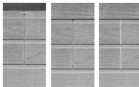
**NOTE:** When using sealant, movement in the planks may result in visible bulging or concaving of the sealant. In some cases, such as where extreme changes in moisture have occurred, the sealant may pull away from the board leaving a crack between the sealant and the board. This movement will not affect the performance or water tightness of the join, though it may be aesthetically displeasing. If this would cause an issue, Weathertex recommends the use of the traditional joiner.
