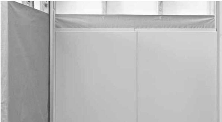
Bring second panel into place and ensure the Self-locking edges of the two panels fully engage. Secure each sheet as per the above fixing detail repeating for all first row sheets. Trim the last sheet to length as required.
