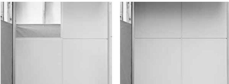
Position the first board of the second row at the corner on top of the board below ensuring the Self-locking edge fully engages. The bottom edge of the second row of Rubix Panels will overhang the top edge of the first row. Fix as per fixing instructions for the first row of panels.
